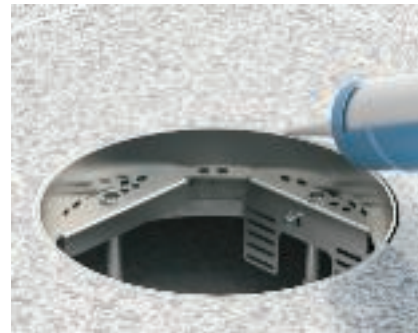
Laying the floor covering on the cassette frames Work the floor covering to the cassette frame. Seal the remaining gap between the floor covering and the cassette with suitable materials.
