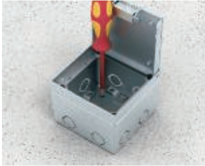
Mounting on the raw ceiling Fasten the installation on the raw ceiling.
