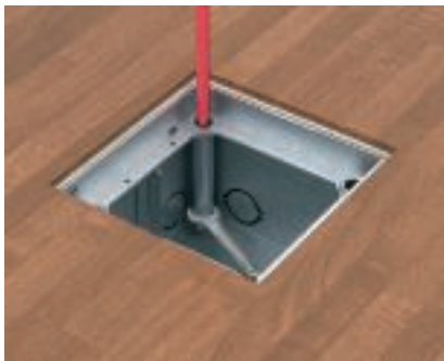
Adjustment to the top edge of the finished floor Adjust the height and lock the height-adjustment screws with locknuts.
