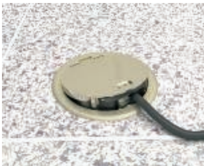
Service outlet with connected connection cable Used service outlet.
