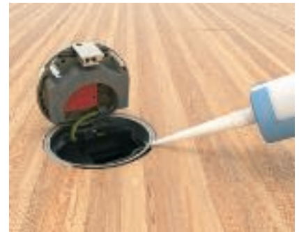
Sealing of service outlet with contact frame Create a seal for the service outlet using a permanently elastic filler (construction work).
