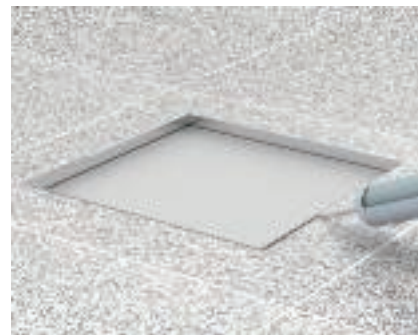
Laying the floor covering on the cassette frames Work the floor covering to the cassette frame. Seal the remaining gap between the floor covering and the cassette frame with suitable materials.
