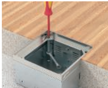
Height adjustment of the UDHome4 The minimum installation depth is 95 mm (measured from the raw screed to the top edge of the screed). The installation unit possesses four interior stable support brackets with a height-adjustment area of up to 30 mm and can thus be adjusted to the level of the finished floor.
