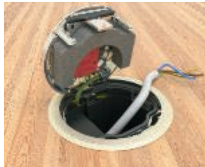
Preparation of socket connection Run the connection cable through the mounting box. Mount the mounting box in the service outlet. Remove the insulation of the connection cable.
