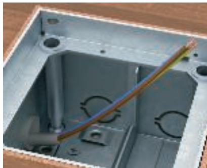
Preparation of connection cable socket Prepare the connection cable for the socket.
