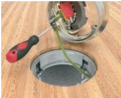
Connection of PE cable Connect the PE connection cable.
