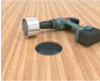
Preparation of mounting opening in system base Create an installation opening of Ø 120 mm. Note: The thickness of the floor structure must be at least 20 mm.
