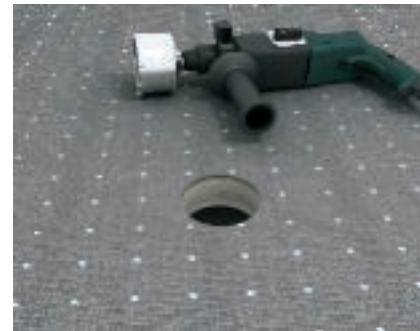
Creation of an installation opening by drilling Create an installation opening with a crown drill.
