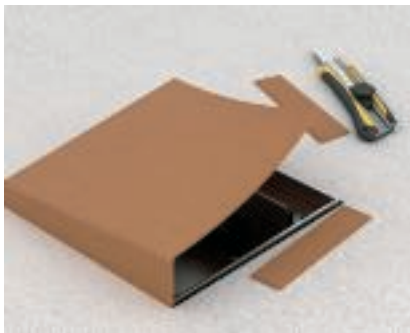
Opening after screed work Open the cardboard cover with a knife and remove the mounting protection lid.
