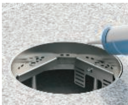
Laying the floor covering on the cassette frames Work the floor covering to the cassette frame. Seal the remaining gap between the floor covering and the cassette with suitable materials.
