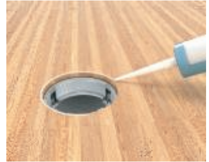
Sealing of service outlet in system base Create a seal for the service outlet using a permanently elastic filler (construction work).
