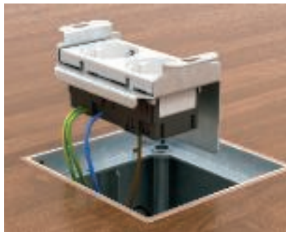
Connection of PE cable Connect the prepared PE cable to the socket.
