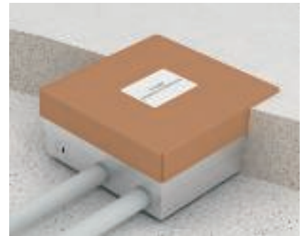
Screed work Lay the screed and work it to the flush-mount unit. Do not use a separating layer.
