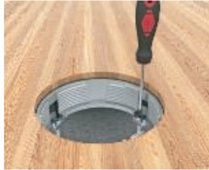
Insert the mounting ring in the system base. Insert the mounting ring in the opening so that it is flush with the top edge of the screed and screw it tight.
